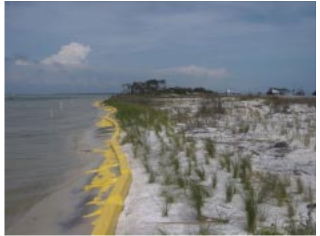
Okaloosa Island after installaion of plants and sediment curtains
